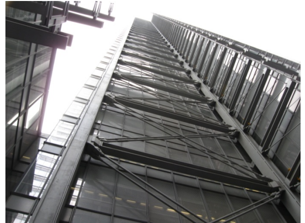
Figure 8: Image of Rod X-Braces at Notches
